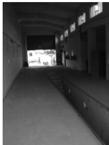
Inspection pit at the Burari inspection centre
